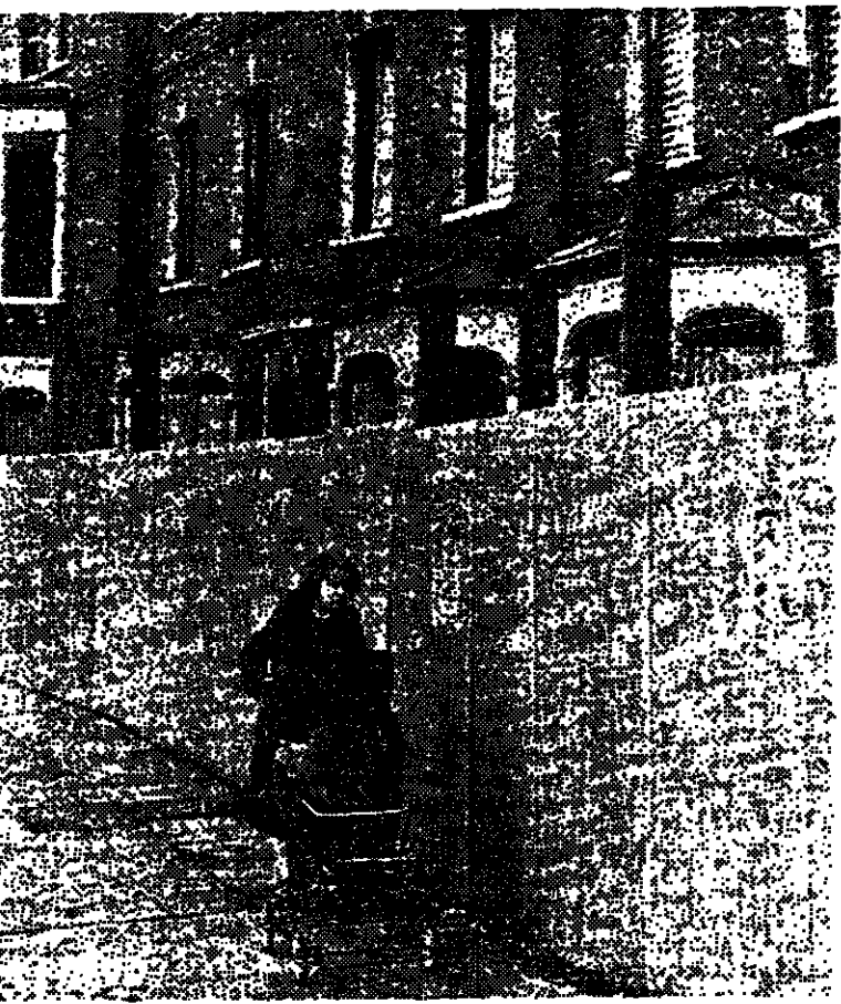
Decay and dereliction, and it can only get worse
